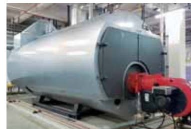
Vitomax HS (13.0 t/h, 10 bar) Customer: PT. B. Braun Pharmaceutical Indonesia
