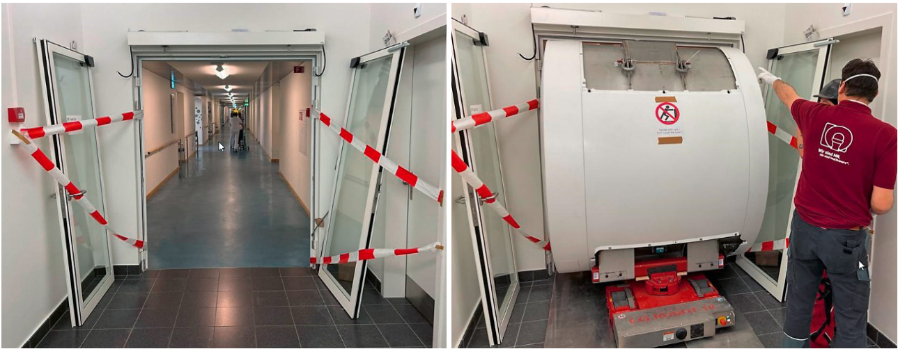
5 MAGNETOM Free.Max installation at University Hospital Basel in Switzerland. Even during one of the very first installations, the small size of the system and the eliminated quench pipe paid off to make the installation process much easier.
