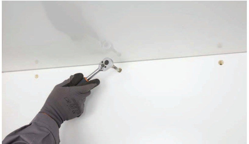
Cold room assembly
