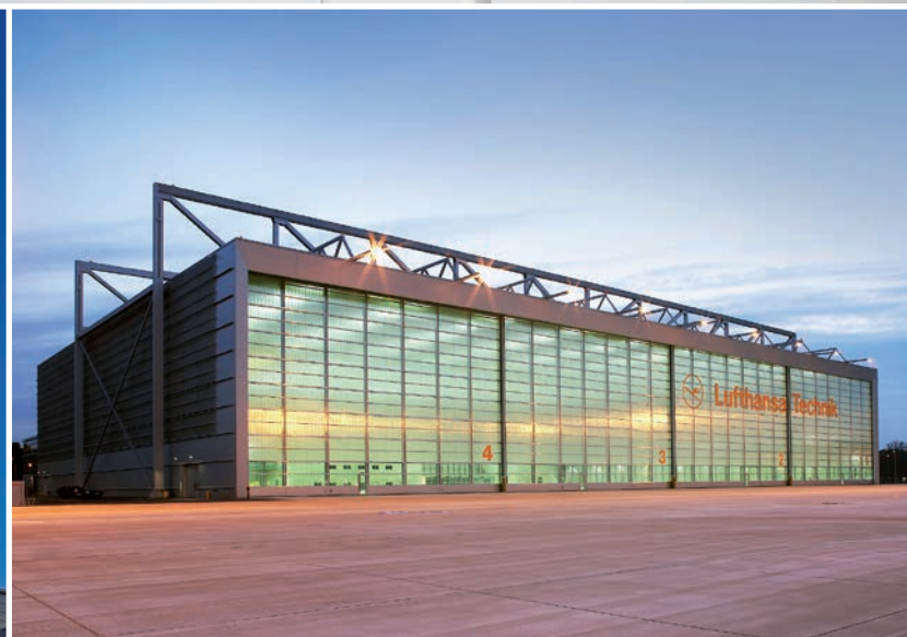
Lufthansa Technik built a dedicated hangar at Frankfurt Airport for the technical servicing of not only the Lufthansa A380 fleet.
